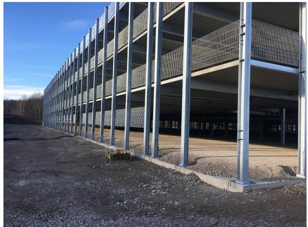
Figure 5: Six-level prefabricated parking structure involving welding and joint sealing. Built by our partner Goldbeck.
