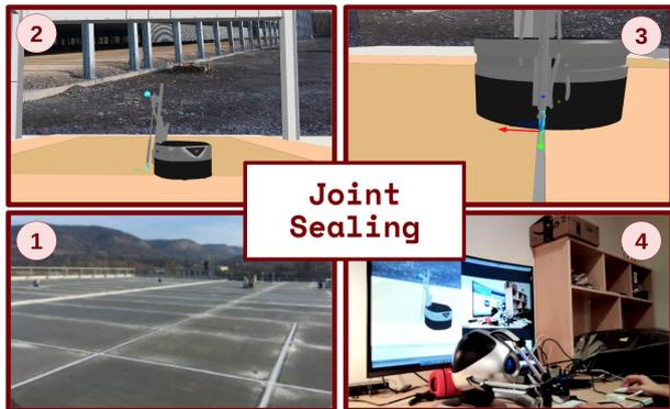
Figure 3: Concrete joint sealing four-step method: (1) collect data, (2) generate simulation environment (3) simulate autonomous behaviors, (4) allow for haptic intervention.
